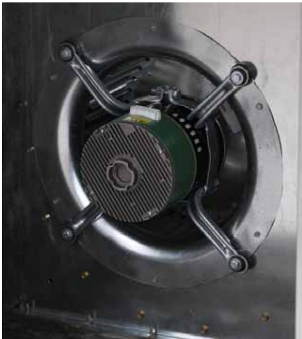
Figure 31. Blower coil with Trane ECM
