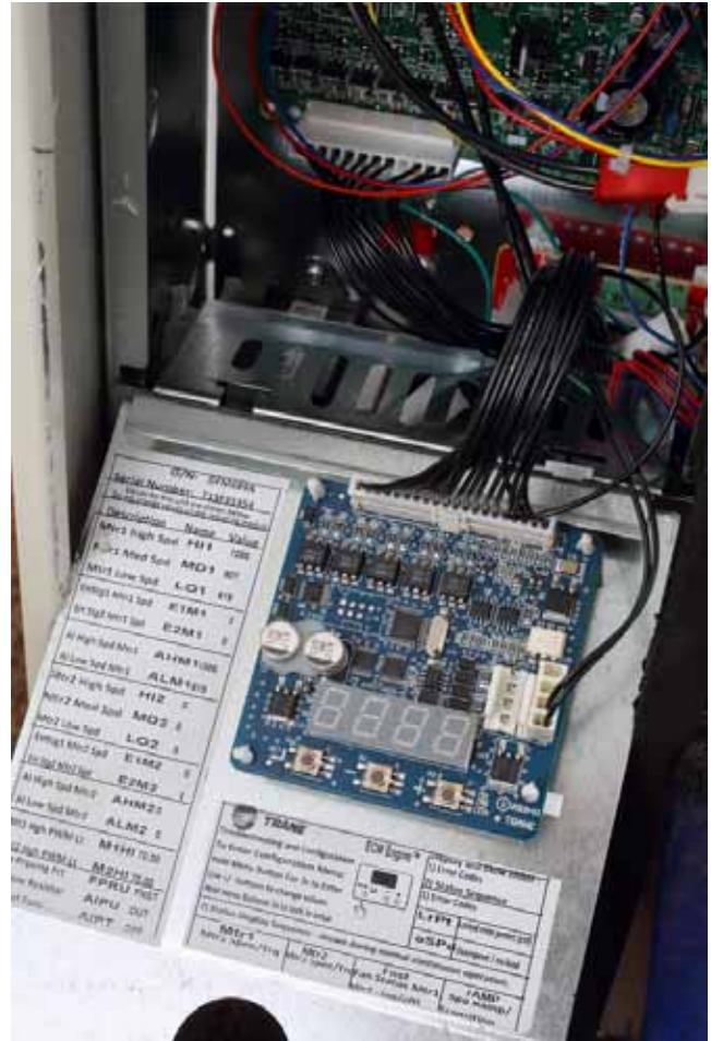
Figure 37. VelociTach motor control board
